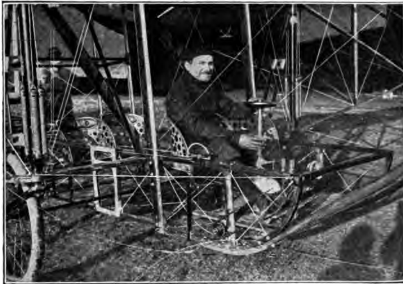
Fig. 14. Close View of Bleriot "Bus," Showing Seats for Passengers
